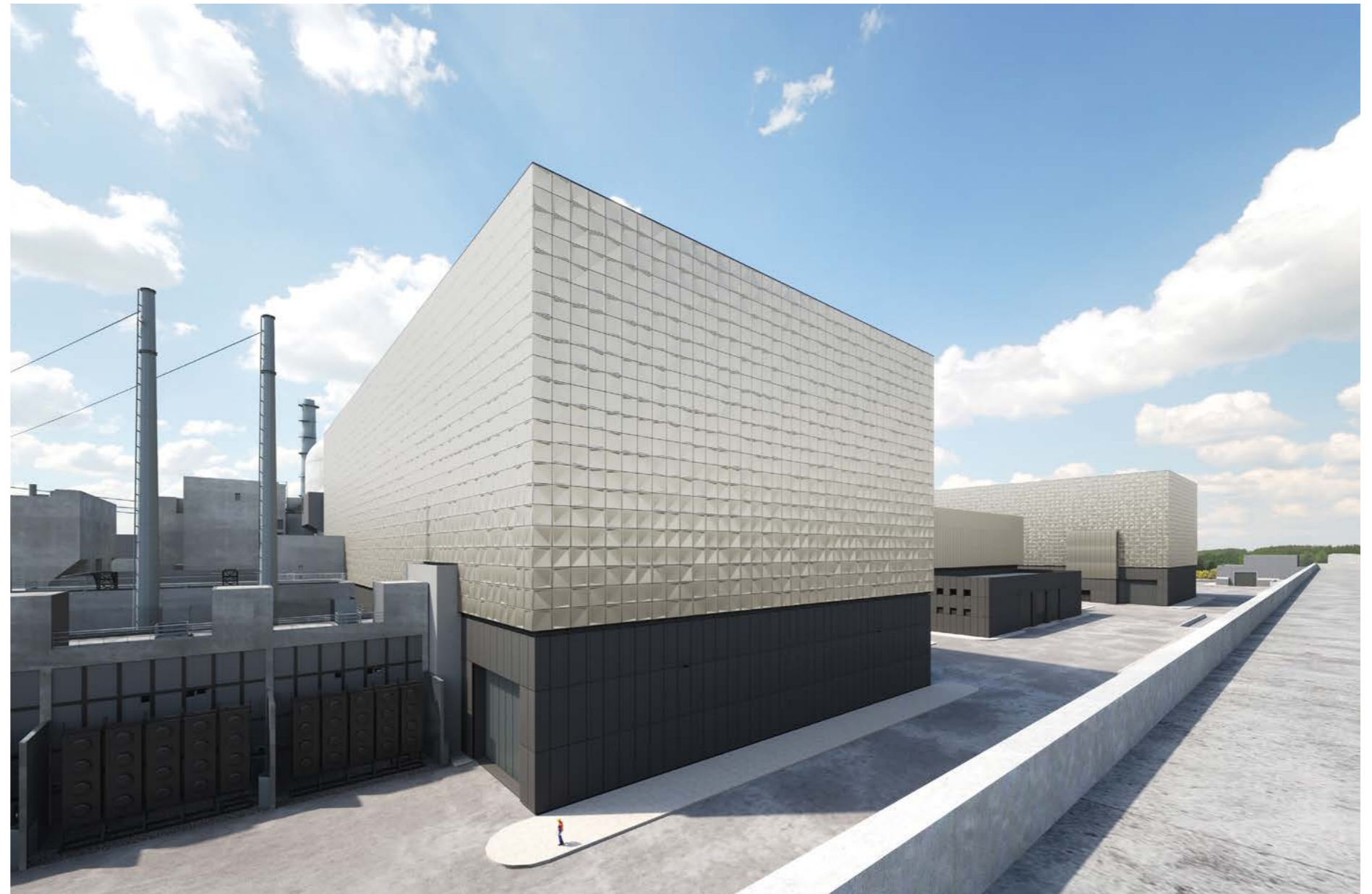
Figure 7.59: View showing the eastern elevation and building sequence of the operational service centre between the turbine halls
