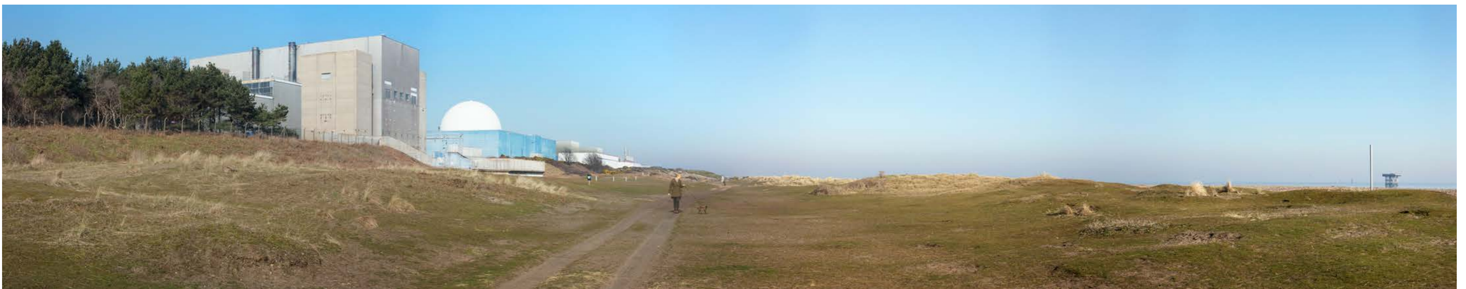
Figure 7.41: Illustrative view north towards the Sizewell C site from the Suffolk Coast Path and Sandlings Walk east of Hill Wood (refer to Figure 13.10.41 of Volume 2, Chapter 13 of the ES , Doc. Ref. 6.3)
